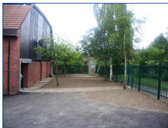
Amy's memorial garden before work began.
