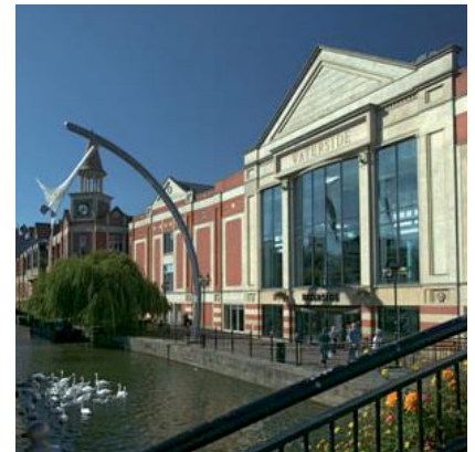
Waterside Shopping Centre, Lincoln
