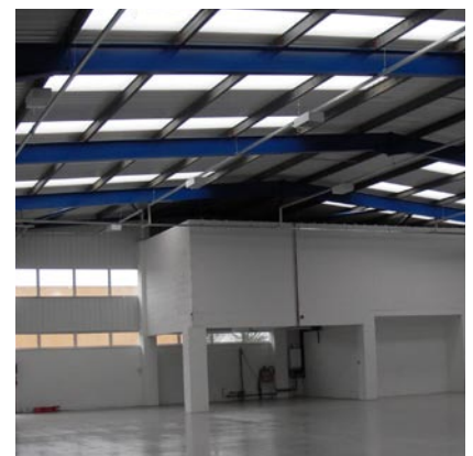
Griffin Industrial Estate, Southampton
